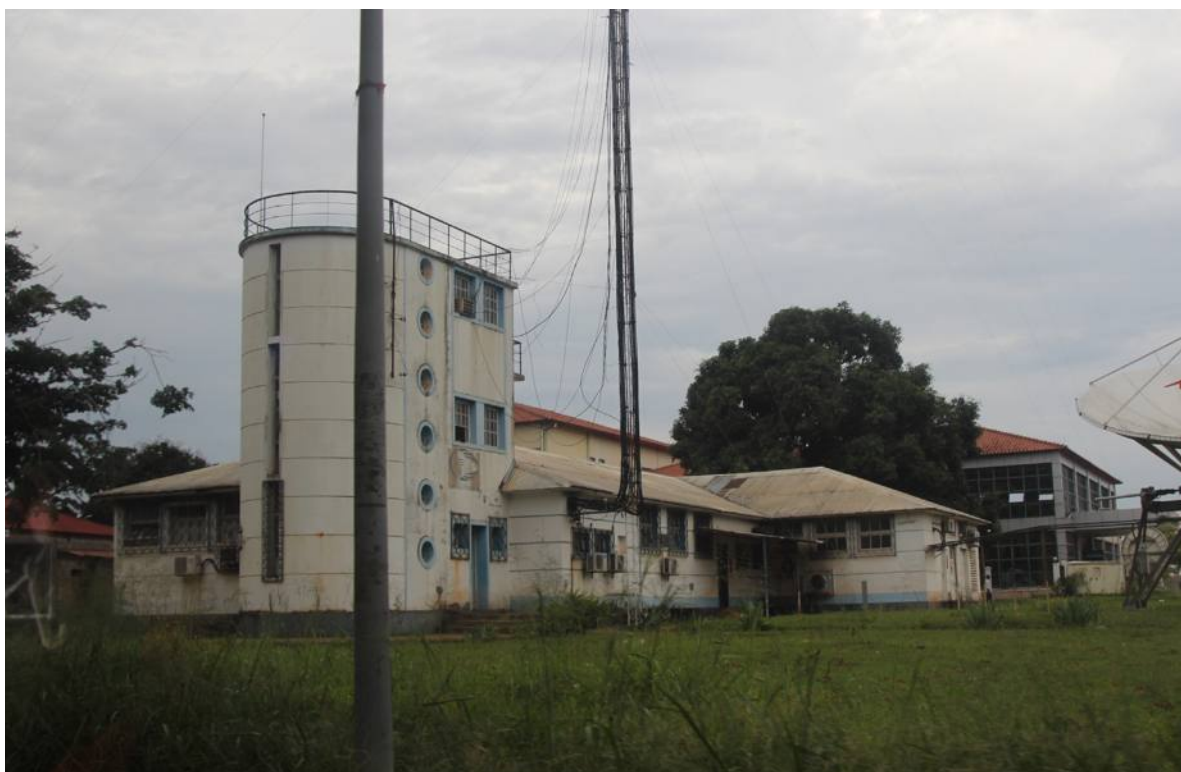
Angola Telecom [Dundo]
