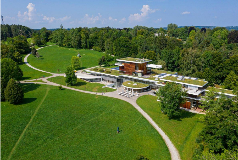
Anexo I- Museu Buchheim in Winkelkötter, C. (s.d.). Filmlocations. Film StarnbergAmmersee. https://www.film-starnbergammersee.de/filmlocations/buchheim-museum-museum
