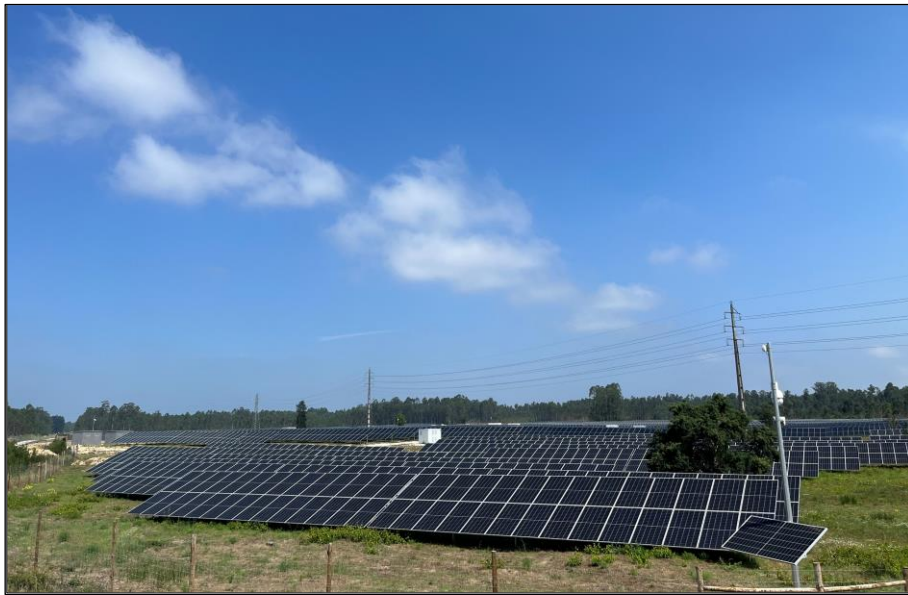
Figure 1.1. Solar power plant - also known as solar park/farm.
