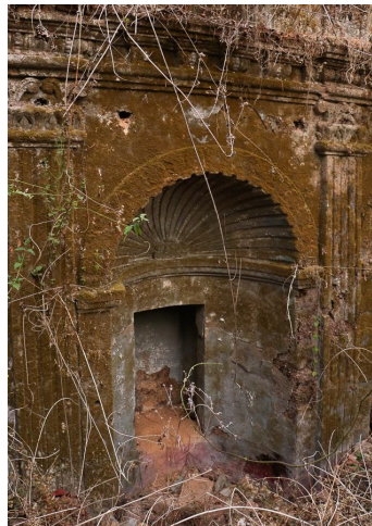
Figure 62: Ruins of an inverted shell niche that survives in the Chapel interior. (Goa: Lester Silvera, 2019)
