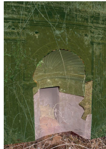
Figure 63: Diagnosis of ruins of an inverted shell niche that survives in the Chapel interior on Fig. 62
