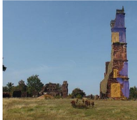
Figure 85 : Diagnosis on façade of the Church on Base Fig. 84
