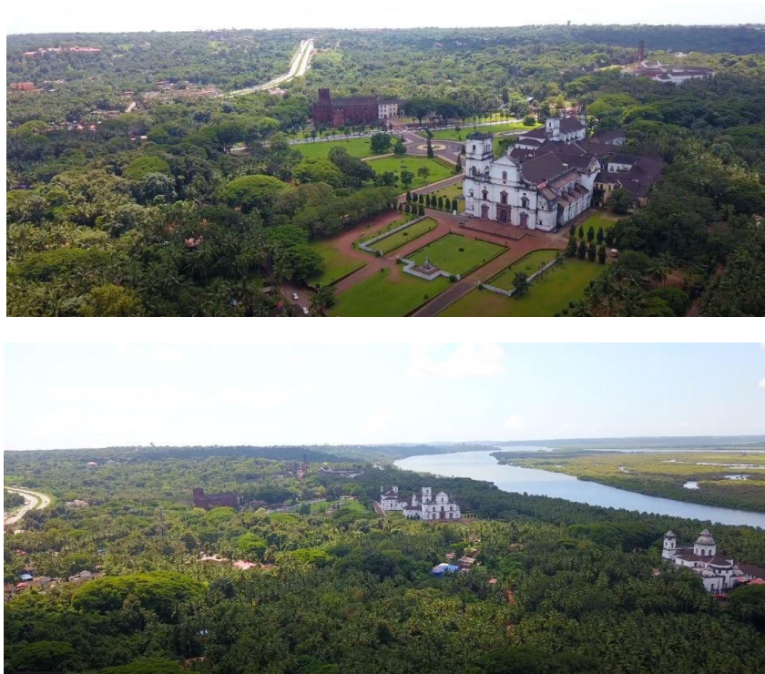
Figure 20: Drone images showing the newly constructed highway (far left) within the buffer zone of the UNESCO protected Heritage sites. (India : 123RF, 2021)
