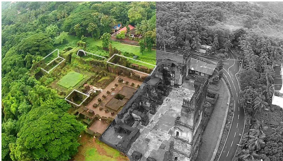
Figure 101 : Zones marked out within the Convent of St. Augustine to recreate the lost volumes and allowing vegetation to grow over the installation as a volumetric guide.
