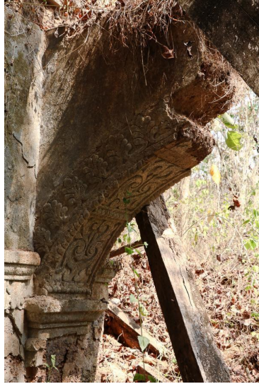
Figure 60 : Stucco patterns on what remains of the arch over the narthex. (Goa: Lester Silvera, 2019)
