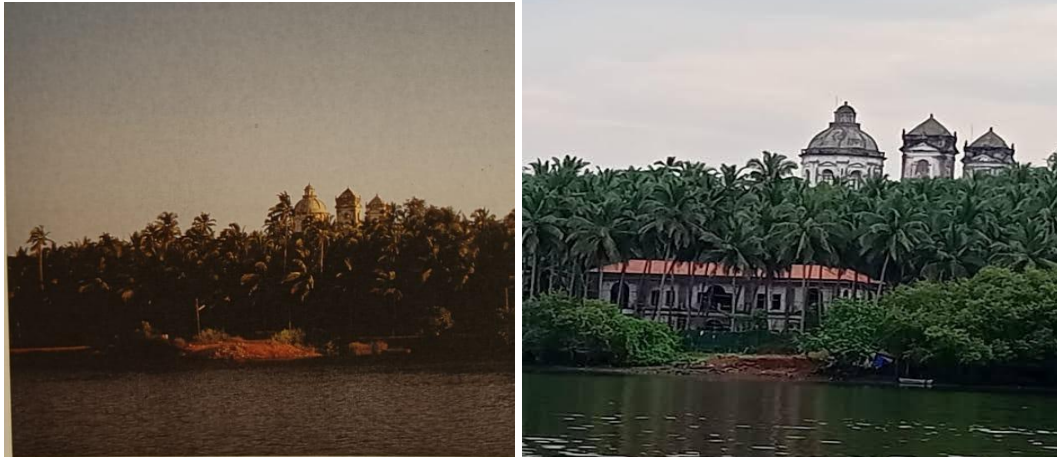
Figure 7: Images from the river Mandovi, to the left by Rossa (1997) and to the right showing the illegal construction by TOI (2021)
