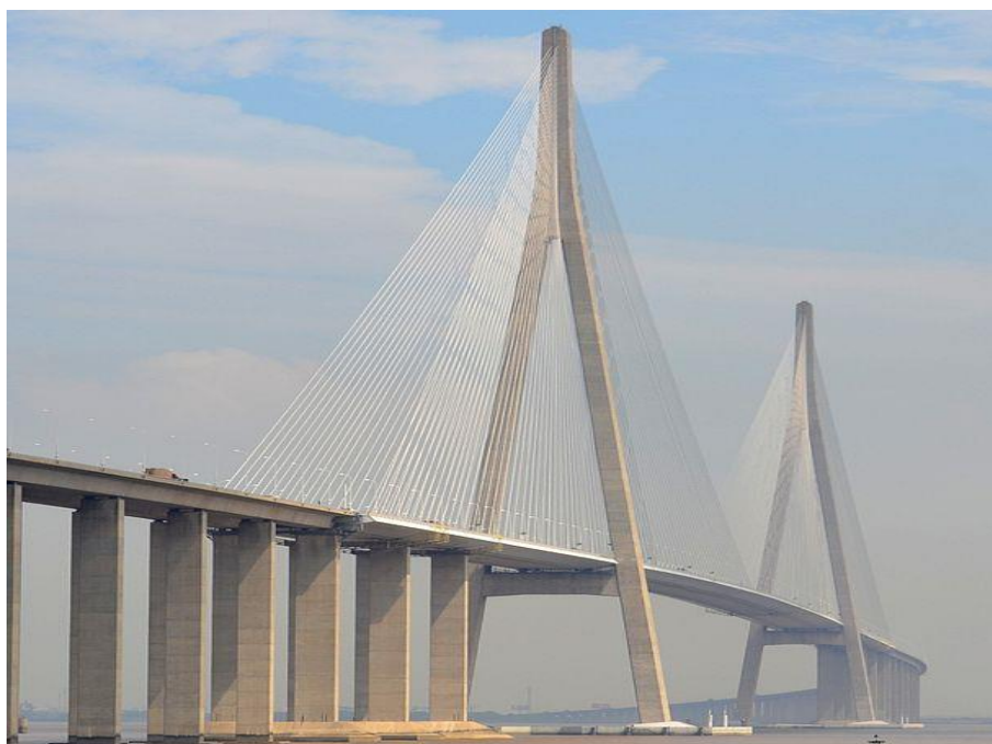
Figure 2.6 – Sutong Bridge (Wikipedia, 2015)
