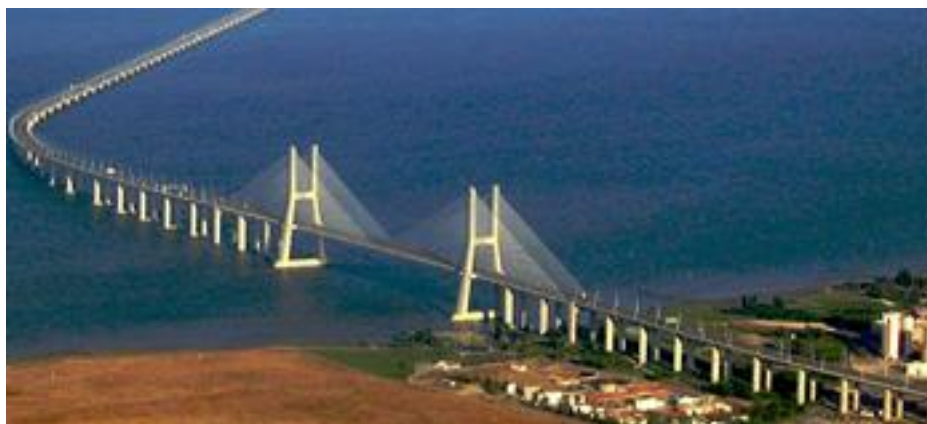
Figure 2.9 – Vasco da Gama Bridge ( http://www.thelisbonconnection.com/ , 2015)
