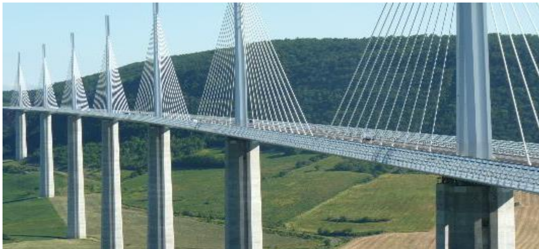
Figure 2.12- Viaduct de Millau ( http://circuitosvip.blogspot.pt/2015/01/viaduto-de-millau-franca.html , 2015)
