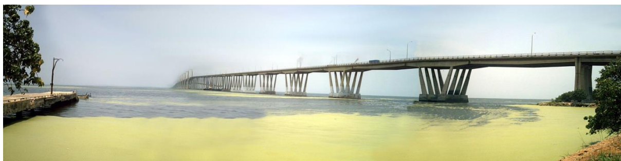
Figure 2.4 - bridge of Lake Maracaibo (Wikipedia, 2015)
