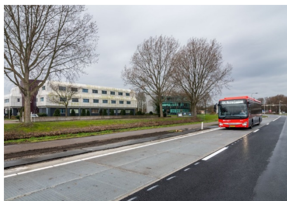
Figure 3. PV pavement product from SolaRoad (Reprint with permission from ref. [21]. Copyright 2019 SolaRoad).
