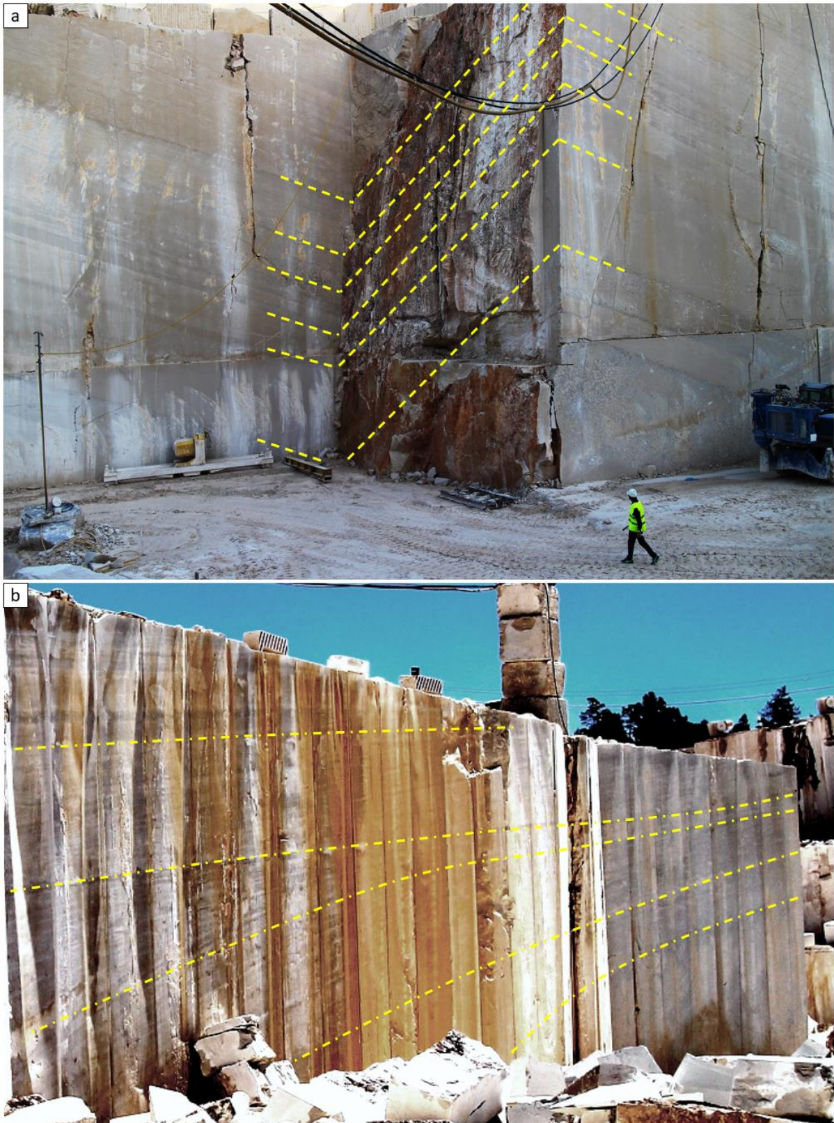
Figure IV.1.8. a : Parallel bedding planes and apparent tabular geometries at Cabeça Veada (Pé da Pedreira Member); b : Prograding/retrograding grainstone bodies at Casal Farto (Pé da Pedreira Member). The height of this front is estimated to be approximately 20 m. Additional detailed interpretations on this quarry front are shown in section IV.1.7.2.1.
