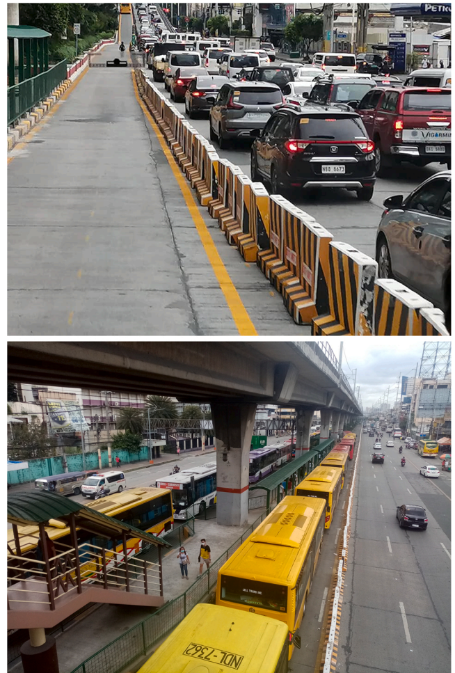
Fig. 8. (a + b). The newly implemented EDSA Busway BRT in Metro Manila. Source: 'Jel' (June 2020); Jack Schmidt (October 2020).
