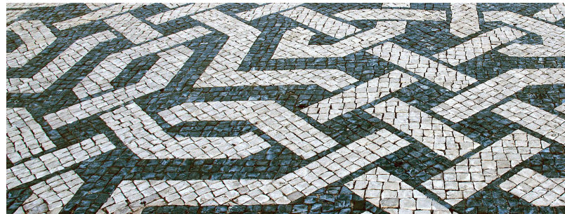
Figure 8. Portuguese pavement in Praça dos Restauradores, in Lisbon.
