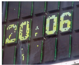
Figure 15. Display with faulty dots.
