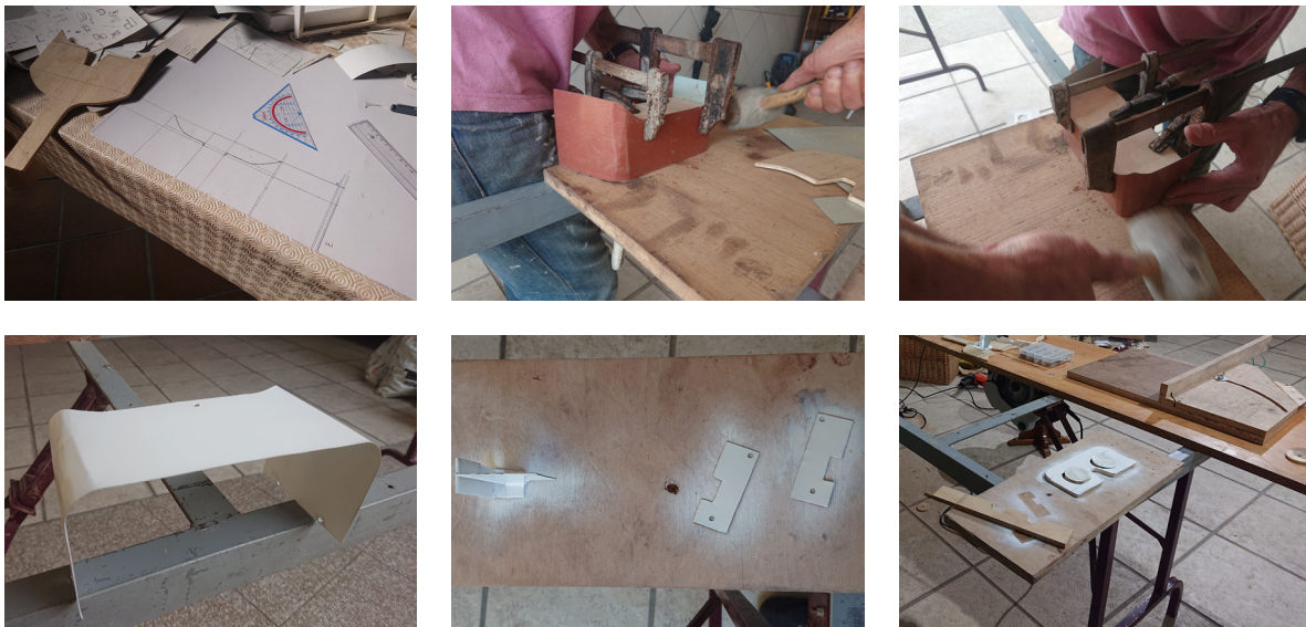
Fig. 106, 107 & 108 (left to right) Top head sheet metal piece building process
