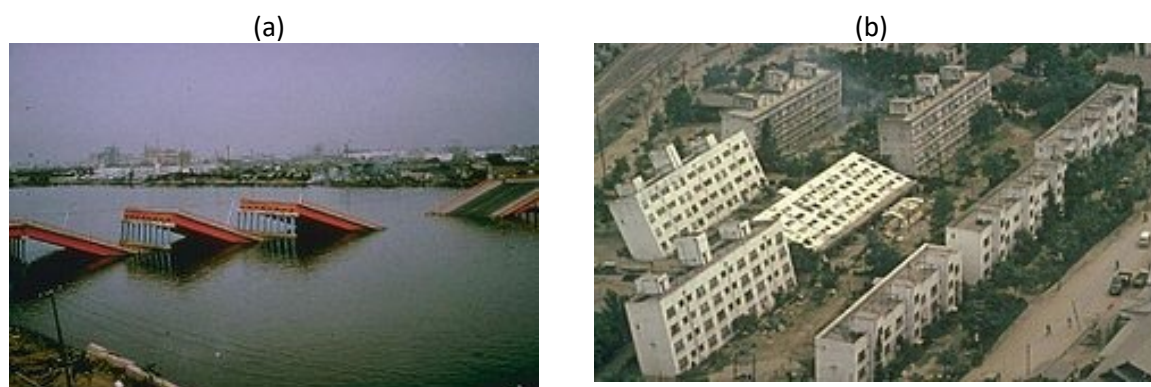
Figure 1.2 – Illustration of liquefaction-induced damage during the 1964 Niigata earthquake (photos from National Geophysical Data Centre, U.S. Department of Commerce): (a) collapse of the Showa Bridge and (b) tilting of Kawagishi-Cho apartment buildings.
