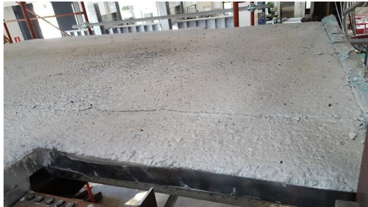
Fig. 5.183 - Collapse of the slab
