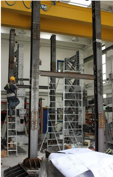
Fig. 5.174 – Columns and beams
