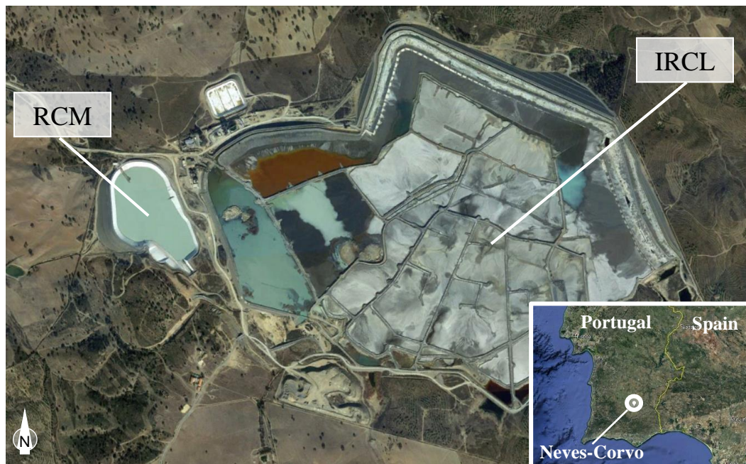
Figure 3.1 - Cerro da Mina Reservoir and Cerro do Lobo Tailings Management Facility (Google Earth, 2020).
