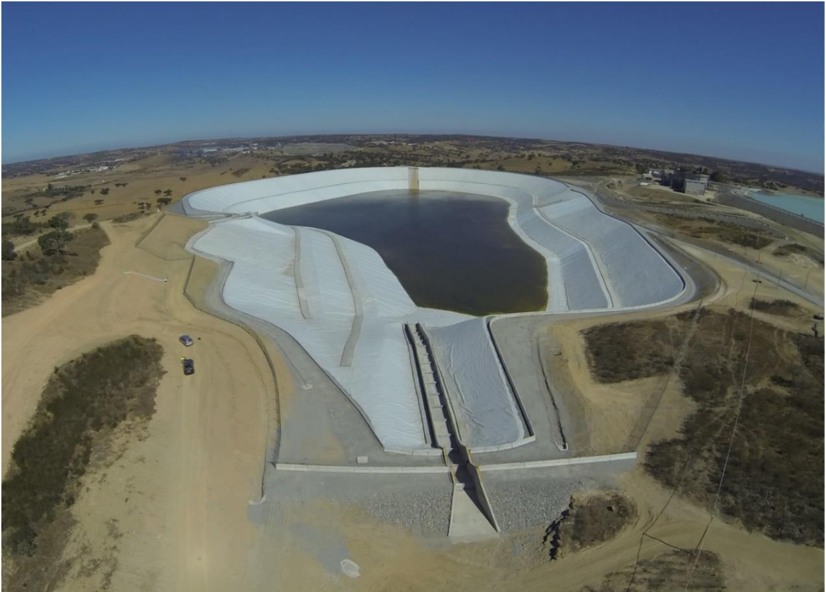
Figure 3.2 - Aerial view of Cerro da Mina Reservoir (Teixeira Duarte, 2010).
