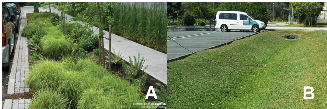
Figure 2.3- Examples of stormwater control measures. (A) bioretention swales- comprised of a filter medium and vegetation, they convey, filter, detain, and even remove nitrogen and other fine particulate contaminants through biological uptake. Source: NACTO (2017). (B) vegetated swales- similar to bioretention swales, with the difference of lacking a filtering medium, and thus not as efficient (Melbourne Water, 2013). Source: Lucke et al. (2014).
