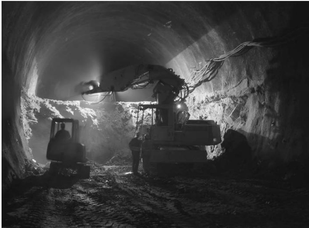
Figure 5- Excavation of the Katschberg Tunnel crown using NATM (Chapman et al., 2017).
