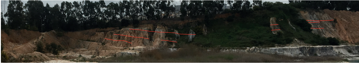
Figure 6.28. South west side of the Via-Vai quarry with bedding planes highlighted. Whole view is 350m.
