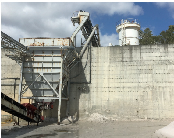
Figure 3.4. Hopper feeding conveyor belt. Reservoir in the background.
