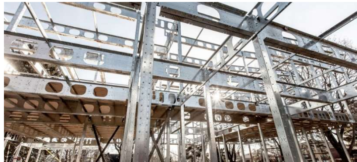
Figure 1.10 - Frame with bolted beam-to-column joists (Bone Structure, 2015)
