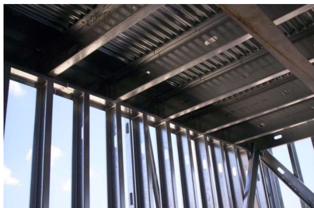
Figure 1.8 - Cold-formed steel floor joists (FDR Engineers, 2019)
