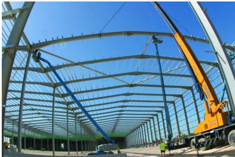
Figure 1.4 - Industrial building roof system (Metsec, 2018)
