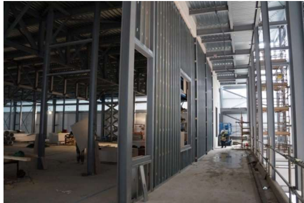
Figure 1.9 - Wall partitions (Steel Formed Sections [SFS], 2018)
