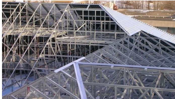
Figure 1.6 - Cold-formed steel trusses (Vanderwal Homes, 2018)
