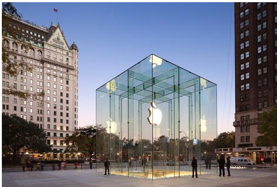
Figure 1.1: Apple Store – 5 th Avenue, New York, 2011 (architecture: Bohlin Cywinski Jackson; structural design: Eckersley O’Callaghan)
