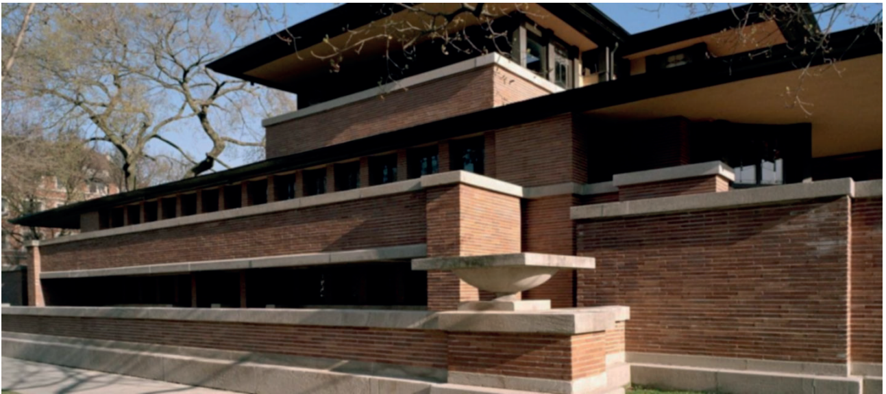
Fig. 204 - Fachada da Robie House de Frank Lloyd Wright.
