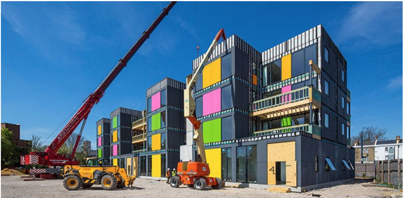
91. CONSTRUCTION OF THE BUILDING, BY STACKING PRE-FABRICATED MODULAR UNITS
