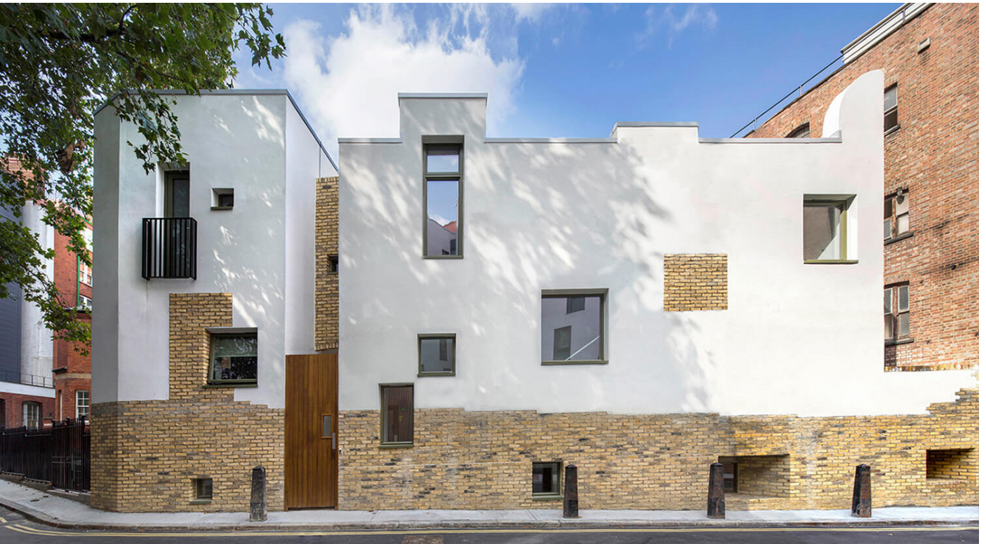
78. MOUNT PLEASANT ELEVATION, STREET SIDE
