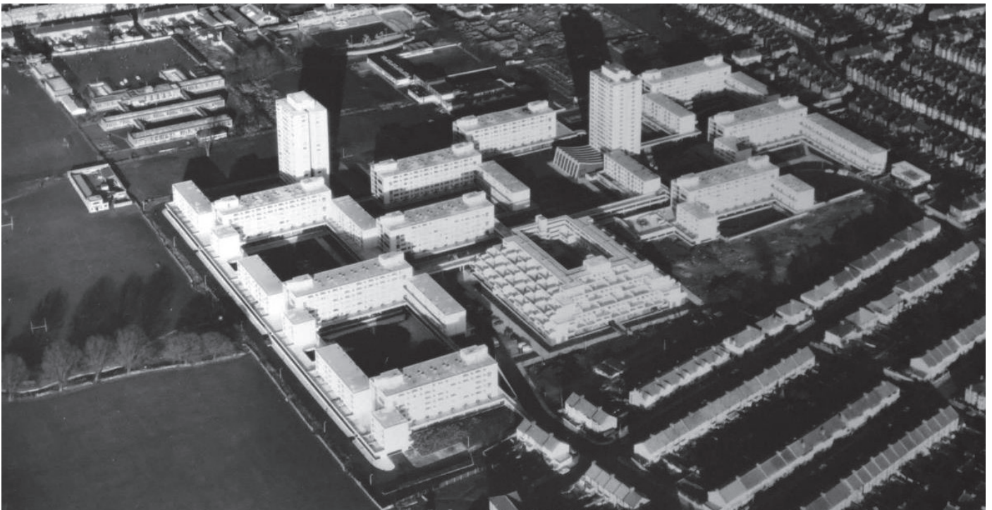
28. HIGH-DENSITY HOUSING IN BROADWATER FARM ESTATE, BUILT IN TOTTENHAM IN 1967
