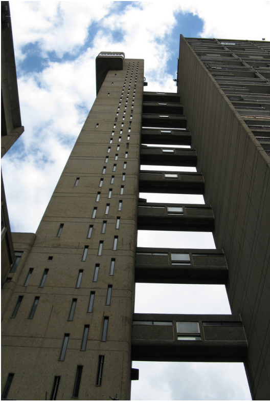
35. TRELICK TOWER - CONNECTION BETWEEN THE TWO TOWERS
