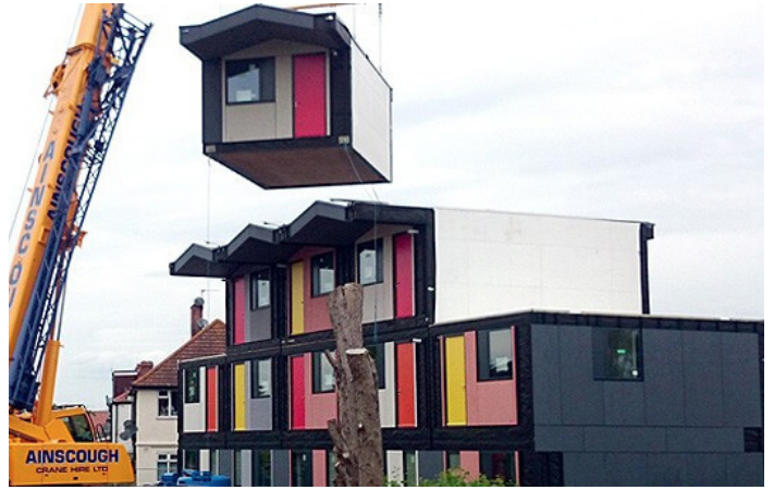
84 AND 85. Y:CUBE MODULAR SYSTEM, MODEL CONCEPT (ON THE LEFT) AND CONSTRUCTION SITE (ON THE RIGHT)
