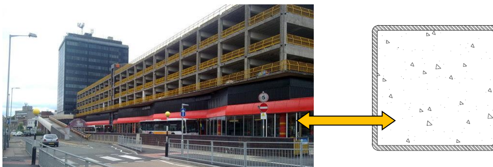
Figura 2.16 - Rochdale Bus Station and Rochdale Municipal Offices. (adaptado de www.geograph.org.uk/photo/2446009 )
