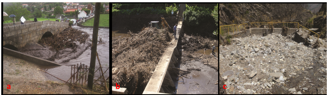
Figure 3. Post-wildfire effects in response to the rainfall episode of 16 th June 2006: a) maximum water level at Pomares Bridge; b) organic and sediment debris blocking the Vide footbridge, Alvoco river; c) regular flow at this season of the year, and sediment deposits after the wildfire in Soita da Ruiva
