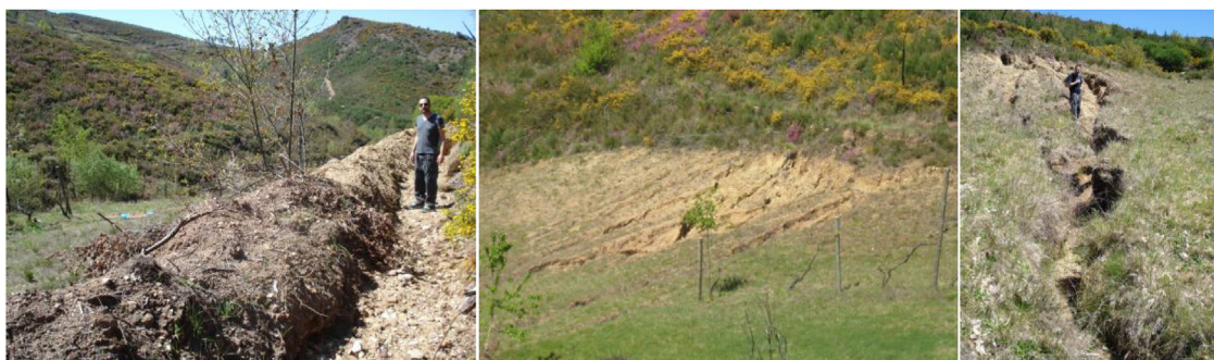
Fig. 2. Seirós runoff water channel (left); view of gullies in July 2016 (centre); a gully detail (right).
