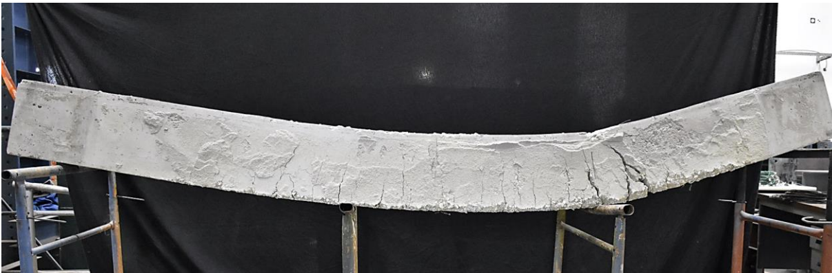
Figure B.4 – Failure mode of the OP-20 beam after fire resistance test
