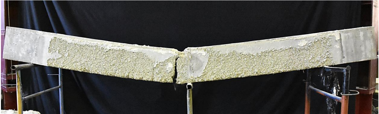
Figure B.6 – Failure mode of the VP-20 beam after fire resistance test
