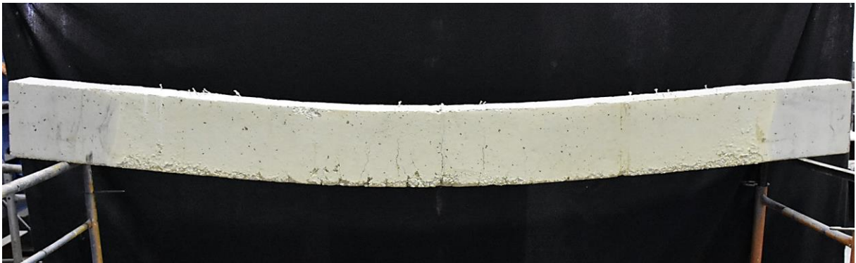
Figure B.1 – Failure mode of the RC beam after fire resistance test (front view)
