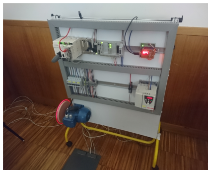
(a) The installation.
