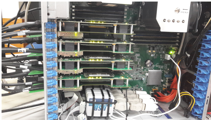
Fig. 3.5 Four Gidel ProceV boards connected to four Terasic USB Blasters through JTAG.
