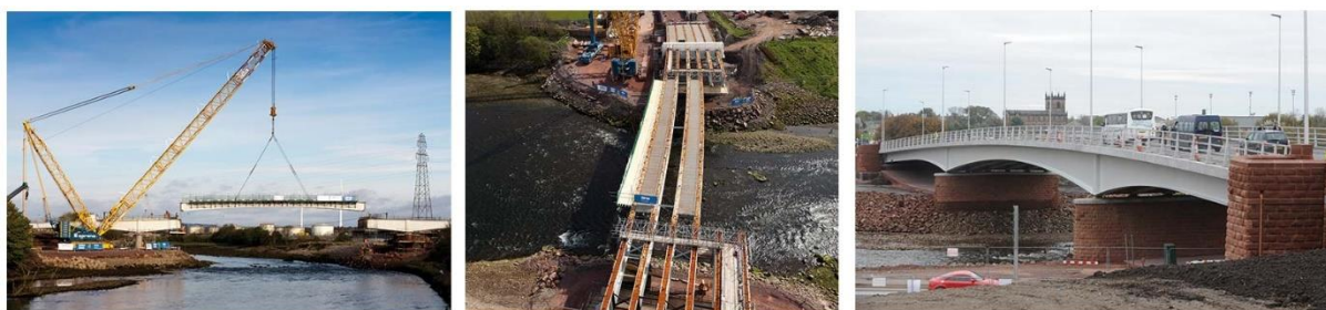
Figura 1.4 – Northside Bridge, Workington (NEWSTEELCONSTRUCTION@2013)
