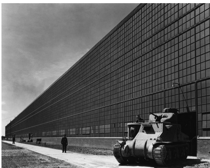
29. Chrysler Tank Arsenal Albert Kahn Associates 1940-42
