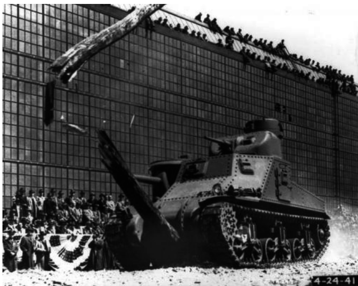
30. Chrysler Tank Arsenal Albert Kahn Associates 1940-42
