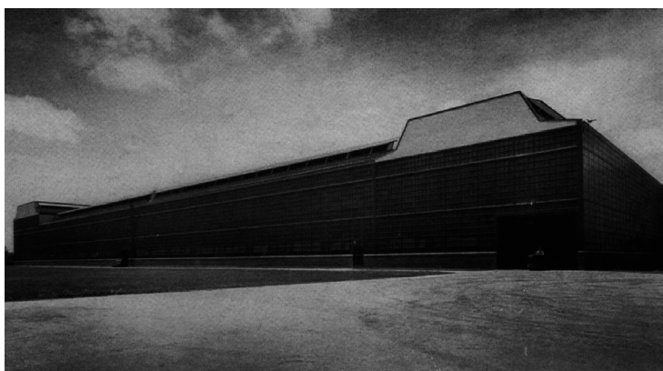
28. Chrysler Tank Arsenal Albert Kahn Associates 1940-42
