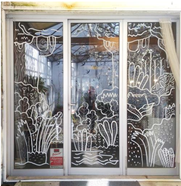
Figure 65 Glass door courtyard
