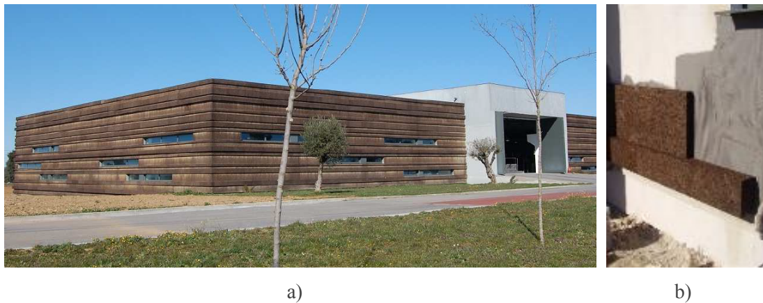
Figure 2-6: Logowines: a) Overview of the building; b) Method of application of the ICB boards.
