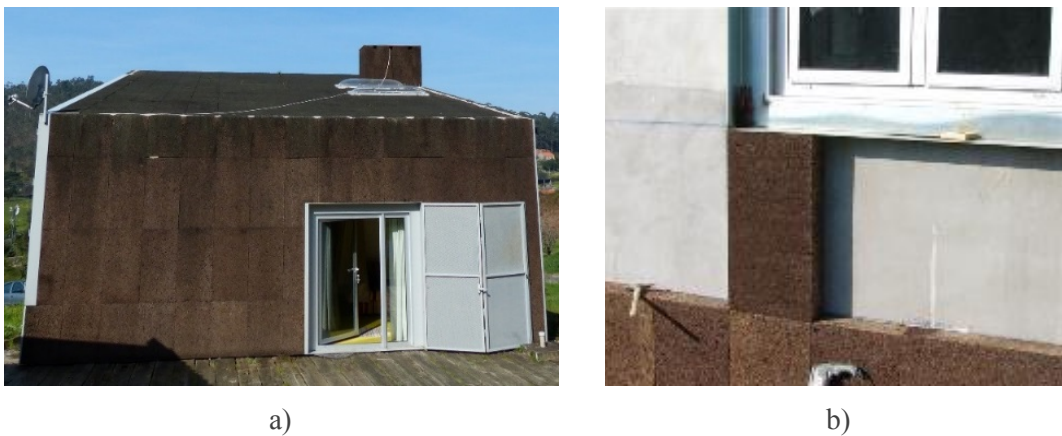
Figure 2-2: Corkhouse: a) Main entrance of the house (view of both facade and roof covered with ICB); b) Application phase of the ICB boards on the concrete walls.
