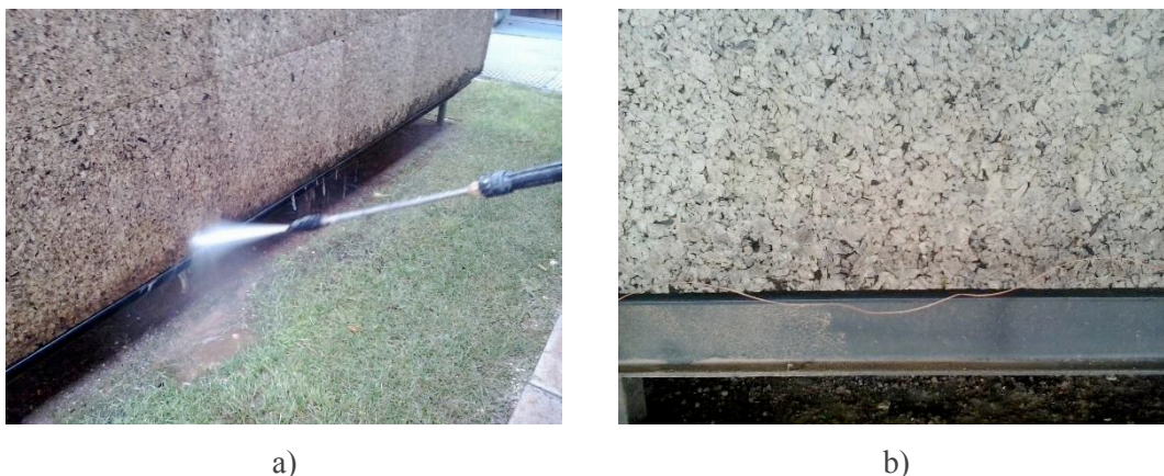
Figure 2-20: Washing of a wall: a) Moss removal with water pressure; b) Facade appearance after being washed.
