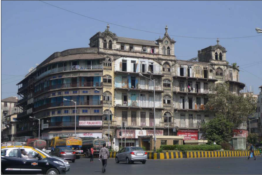
Photo 1. Jer Mahal Building
