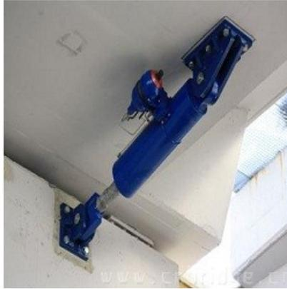
Figura 1.4: Viscous fluid damper
