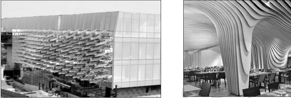
Fig.3,4 Cornell University's Gates Hall, Morphosis - Hinman Research Building Herzog & De Meuron
