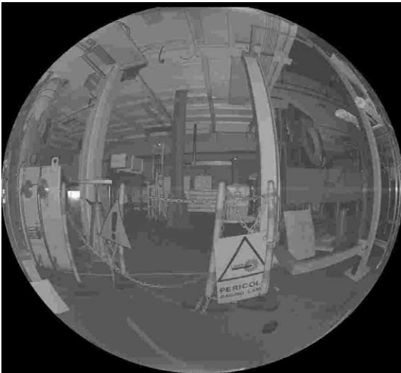
Fig. 4. North view image acquired in a complete scan of the interior of a building.
