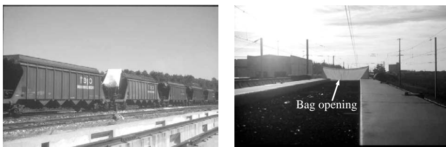
Fig. 8. Rear and front views of the large dust collector installed (left—train in movement; right—train at a stop).
