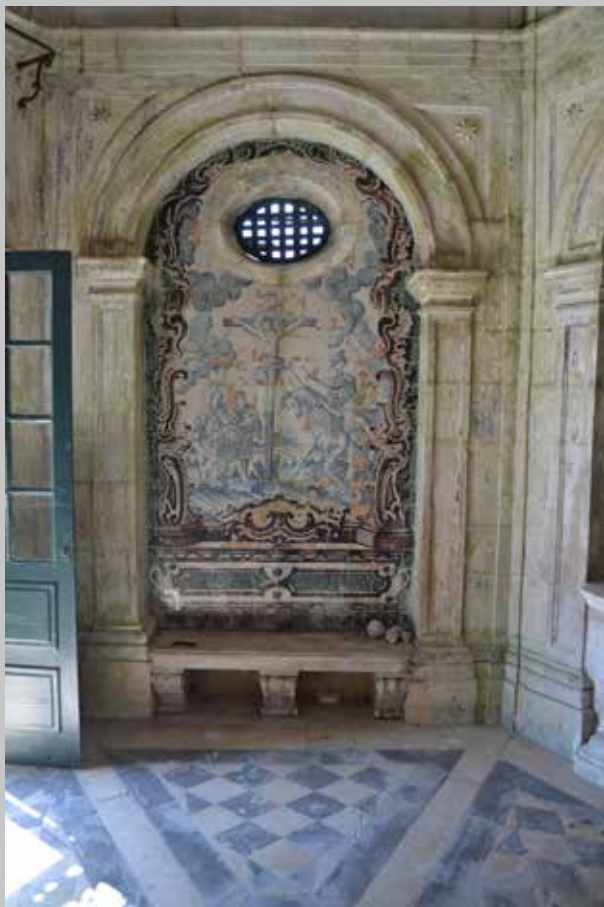
Fig 2. Inside view: filled in arch
