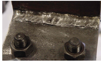
(ii) Detail of the typical crack (WT1a).
