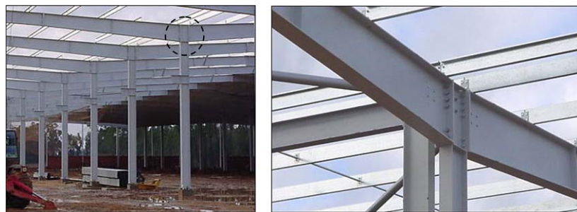
Fig. 1. Example of a pitched-roof portal frame joint.
