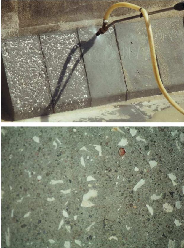
Fig. 5. Substrate surface treated with sand-blasting.
