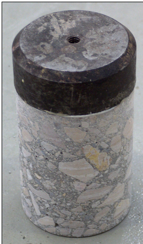
Fig. 6. Pull-off test adhesive failure.
