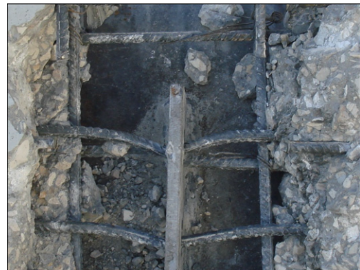
Fig. 14. T-Perfobond connector failure modes with reinforcement bars in the connector holes (TP-2F-120-AR-B).
