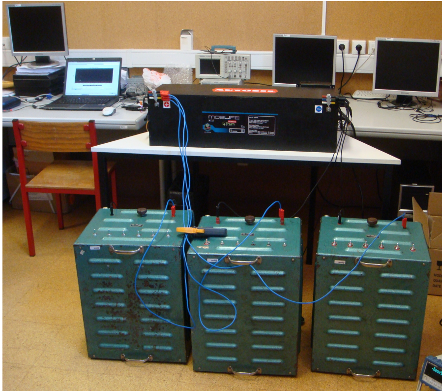
Figure 3.5: Battery test setup.
