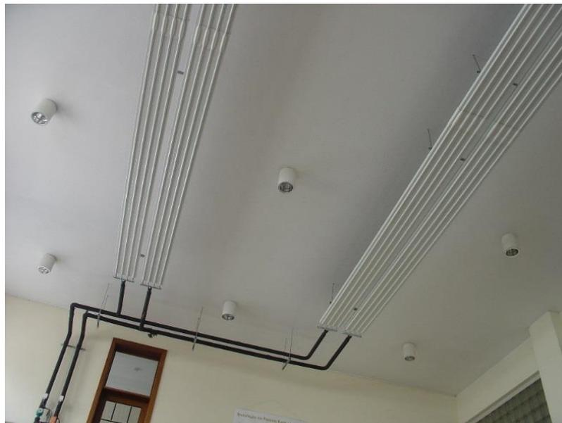
**Figure 1.14.** The radiant ceiling panel circuit of the experimental activity.
