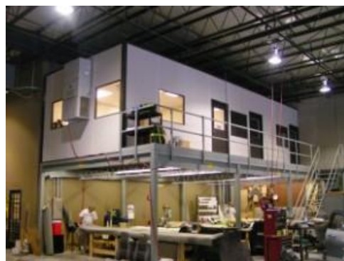
Figure 4.1 - Mezzanine floor inside the industrial building (PortaFab Inplant Offices, 2014)
