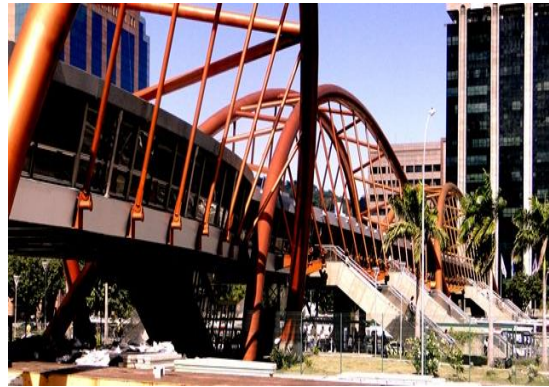
Railway bridge for metro station "Cidade Nova", Rio de Janeiro (CAU/RJ, 2015)
