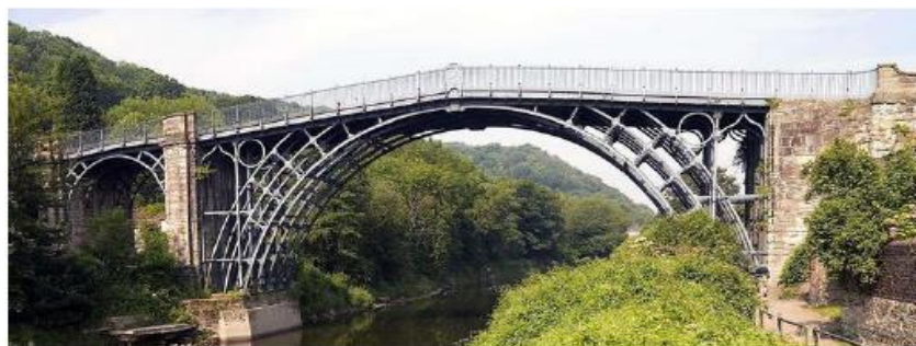
Figure 1.4 - Iron Bridge (English Heritage, 2015)
