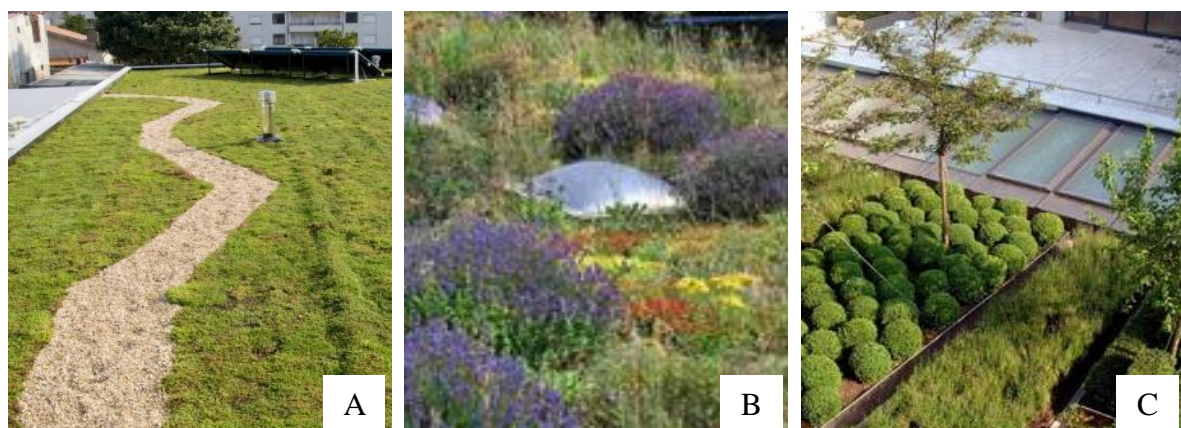
Figure 2.8 - Different types of green roofs. (A) extensive green roof (Neoturf@, 2015); (B) simple-intensive (IGRA (a), 2015) ; (C) intensive green roof (IGRA (b), 2015).
