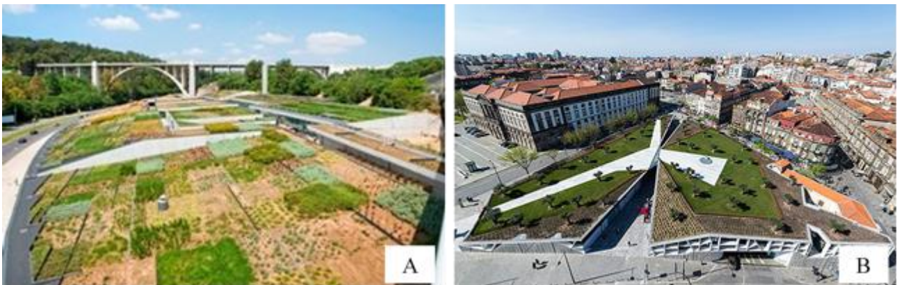
Figure 1.1 - Examples of green roofs in Portugal. (A) ETAR of Alcântara, Lisbon (OE@, 2015); (B) Praça de Lisboa, OPorto (Blog@, 2015).
