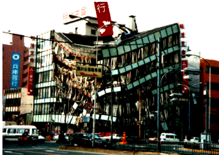
Figure 1.1- Example of the destructive effects of seismic events on building (Great Hashin Earthquake - Kobe, Japan, 1995
