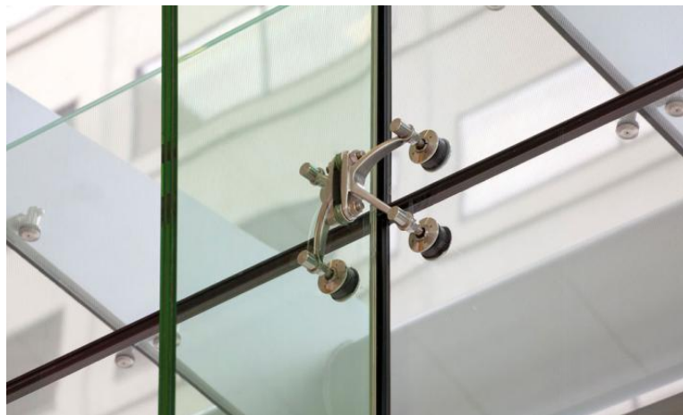
Figure 4 – Spider connector for bolted supports
