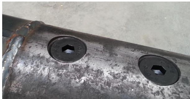
Figure 3.1 – Bolt appearance in connection
