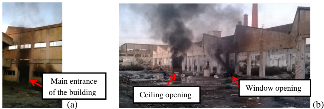
Figure 31- Smoke evacuation: (a) Building main door; (b) Compartment ceiling
